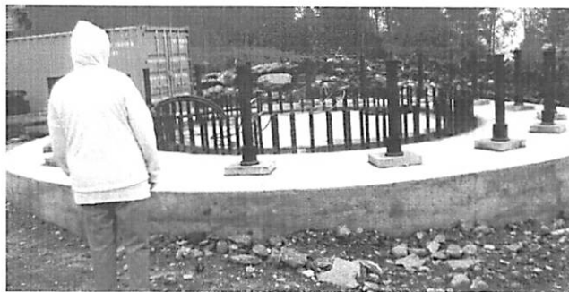
One of the first tower concrete bases to be poured, showing the huge number of anchor bolts required. The double ring inside holds down tower bottom section
